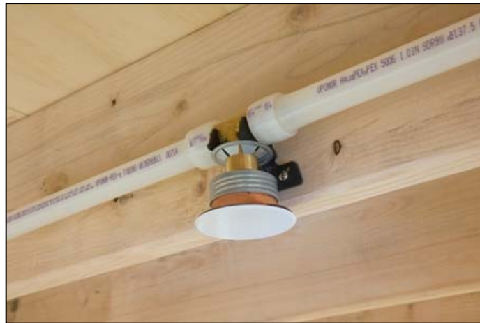
The new ProPEX® Lead-free Brass Fire Sprinkler Adapter from Uponor is a more cost-effective alternative to stainless-steel adapters and provides easier installation on a variety of mounting surfaces.
