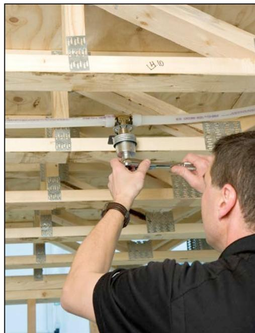
**Uponor ProPEX® engineered polymer (EP) fittings, lead-free (LF) brass sweat and threaded adapters, and Uponor AquaPEX® tubing up to 2" are now listed to UL 1821 and ULC/ORD-C199P for use in residential multipurpose fire sprinkler systems.**
