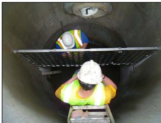
The SAFL Baffle, developed out of the University of Minnesota College of Science and Engineering's St. Anthony Falls Laboratory (SAFL), keeps sediment pollution out of lakes, rivers and oceans.
