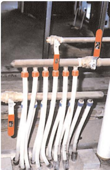
Uponor manifolds supply hot and cold water to fixtures in over 300 units of a residential high rise.
